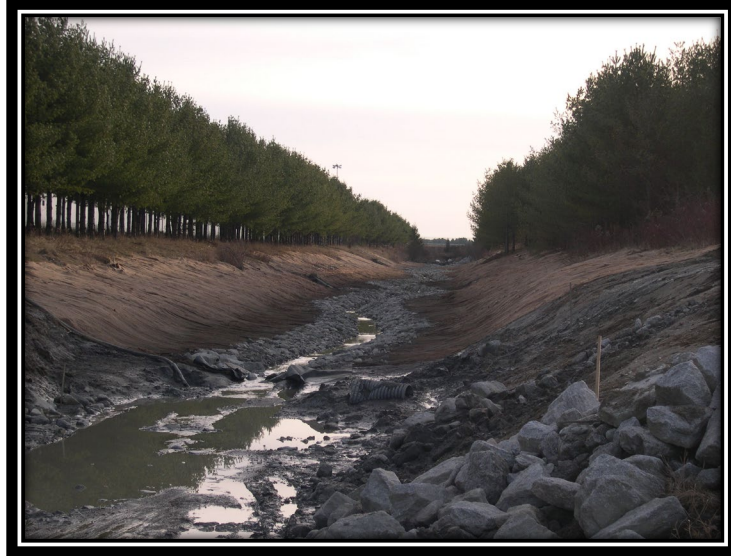
Bangor – Stormwater Management Swale
